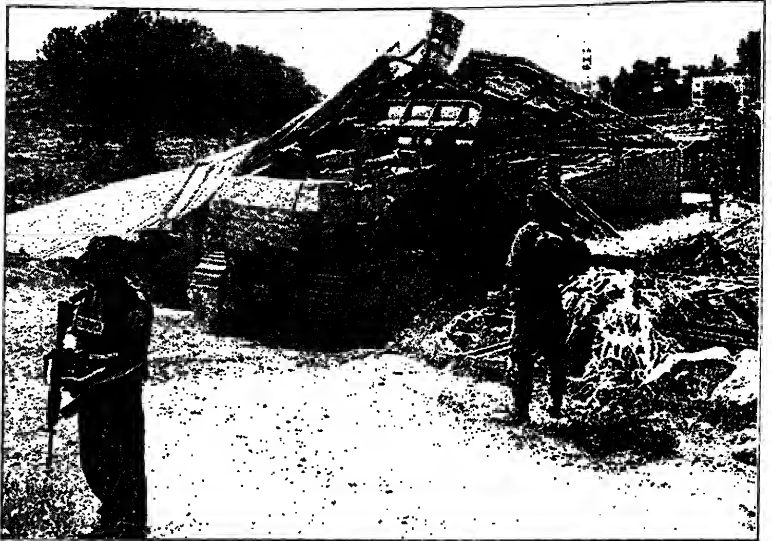
Border policemen stand guard yesterday, as a bulldozer demolishes an illegally built Palestinian home on the outskirts of Hebron. (AP)
